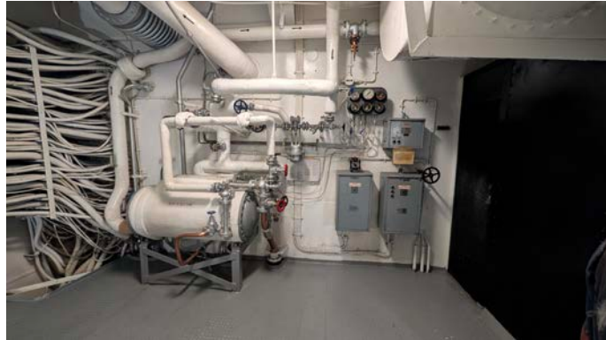
Figure 2 SSTG 1 Air Ejector
